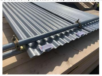
5. Close up of sheet between top and lower tubes
