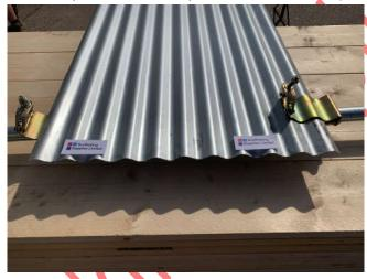
3. Add additional sheets, adding couplers along the lower tube length until the roof area is covered
