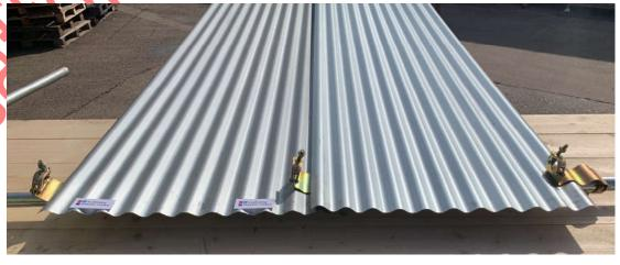
4. Once the sheets are in place, attach the top tube to the couplers, this will "trap "the sheets in place.
