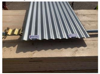
2. Offer the sheet up to the first coupler, then attach the next coupler against the sheet
